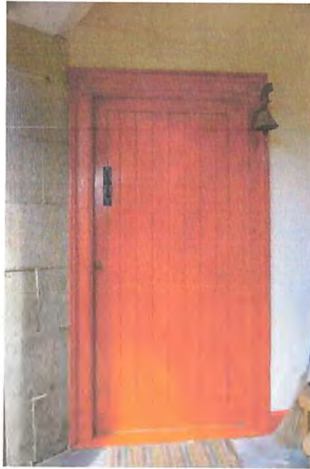
Fig. 30 External view of door GD.01 from Porch to Living Room. This is a replacement door in the original frame and surround.
