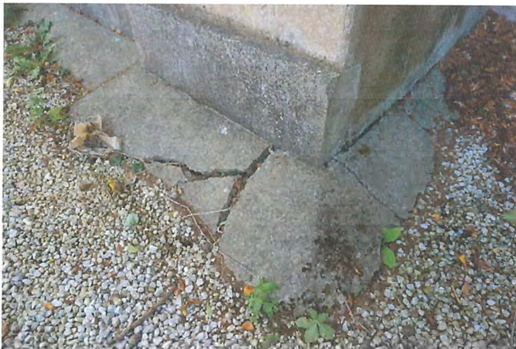
Fig. 39 View of concrete haunching to plinth at north east corner. Note cracking.
