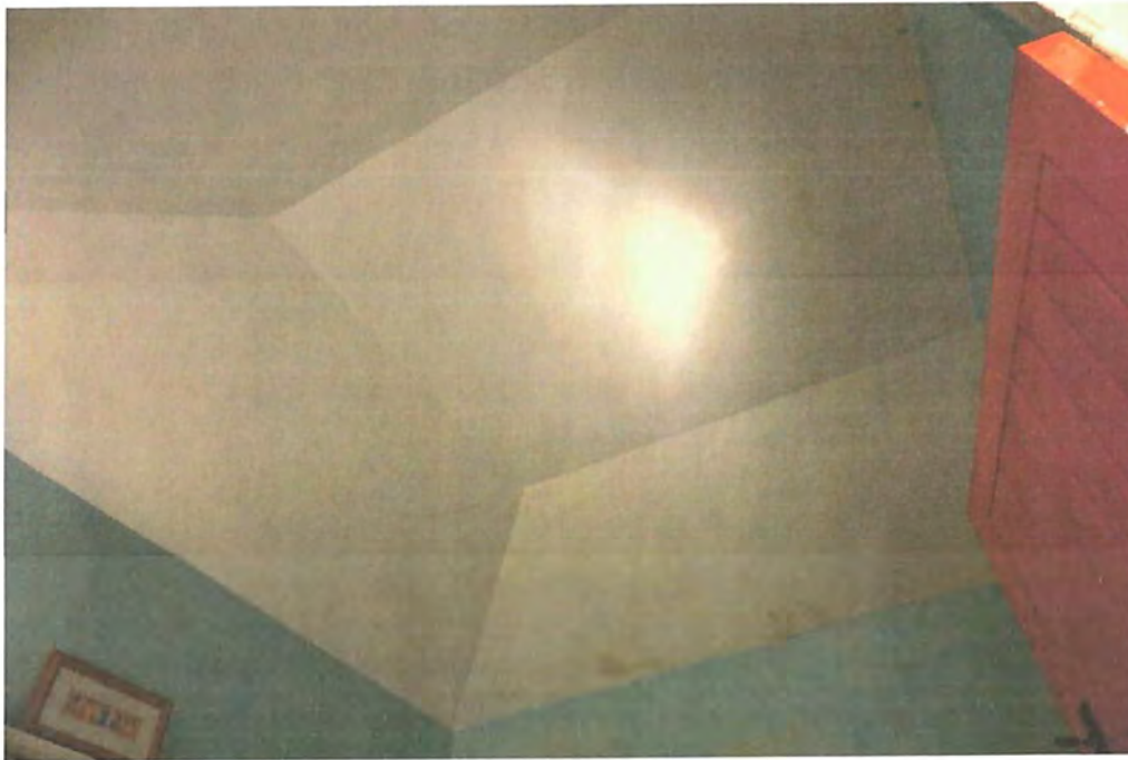
Fig. 28 View of ceiling to GF.01, Living Room. Note staining caused by water ingress.
