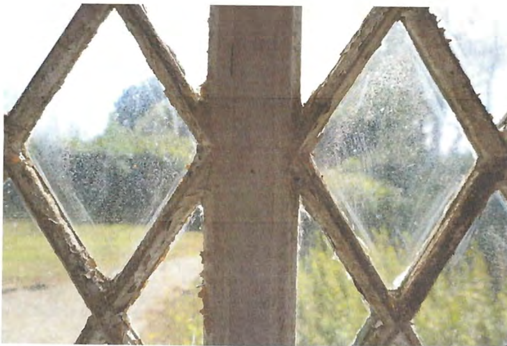
Fig. 22 Detail of lattice glazing.
