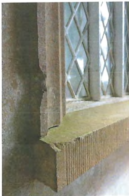
Fig. 25 Example of minor damage to edge of window surrounds at GW.01.
