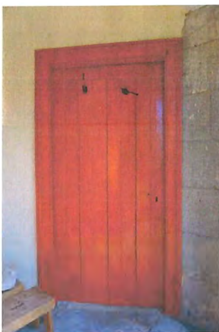
Fig. 32 External view of original door GD.02 from Porch to Bedroom. Note this door is painted shut.
