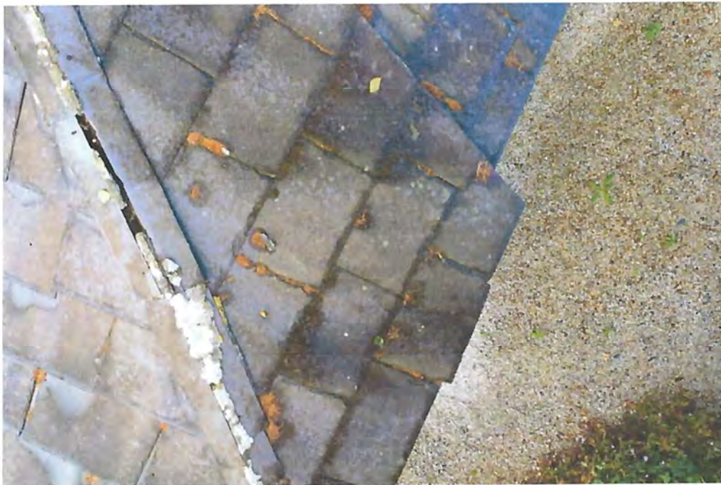
Fig. 16 Detail of roof. Note damage to hipped ridge and instances of slipped slates.
