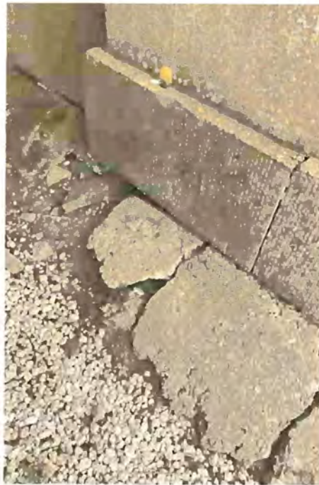
Fig. 38 View of concrete haunching to plinth at the west facade. Note cracking and material falling away from supporting ashlar plinth.
