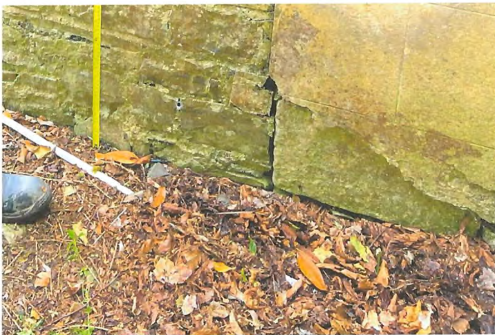
Fig. 37 Example of damage to render on the north facade.
