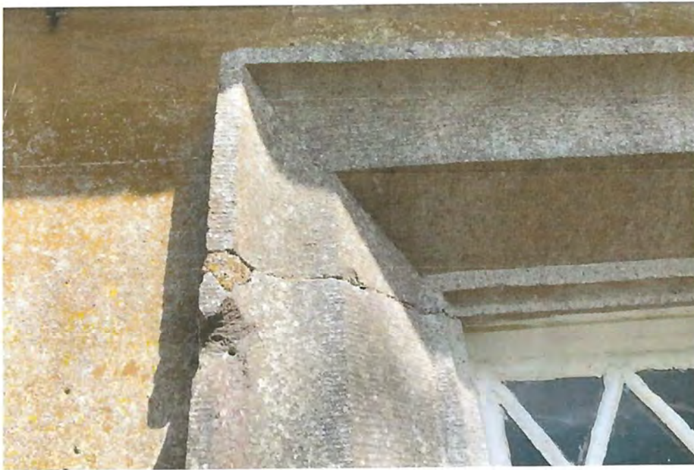
Fig. 24 Example of minor damage to edge of window surrounds at GW.02.
