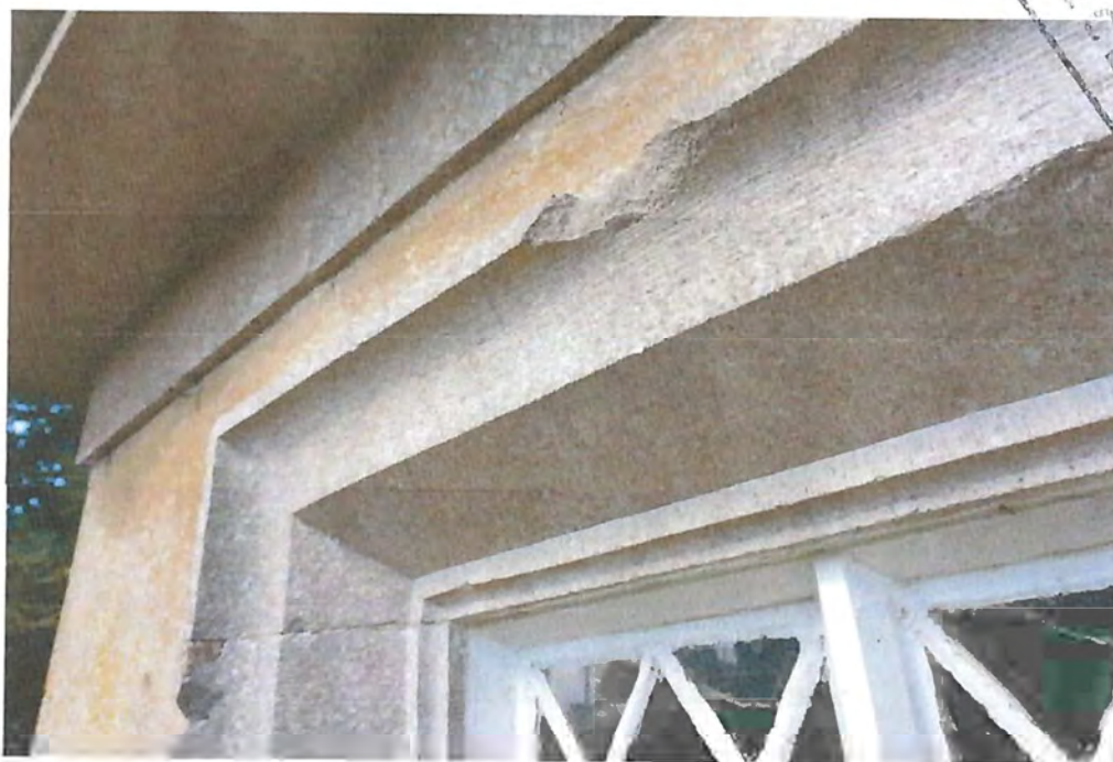
Fig. 23 Example of minor damage to edge of window surrounds at GW.02.
